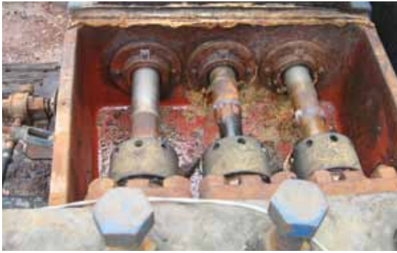
Plunger pumps (shown) have maintenance, wear, lubrication, and environmental issues that Hydra-Cell pumps avoid because of its seal-less, multiple-diaphragm design.
